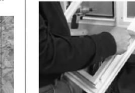
When installing windows next to each other, the outside trim pieces will need to be trimmed to obtain proper fit. A rib is molded into the back side of the trim piece for guiding the cut. Detailed pictures, cut diagrams and mulling videos can be found at the end of the instructions and on the website.
