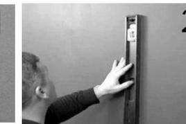
Draw vertical lines using a long level that will locate each edge of the studs. Also draw a horizontal level line for the bottom of the window. The horizontal line should be 2" above where you want the bottom of the Inside Trim to be.
