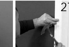
Secure Interior Trim piece with finish nails supplied. Repeat for other windows if multiple installation.
