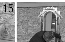
Starting at the bottom of the window, place flashing tape over mounting flange and secure to sheathing. Work vertically until all flanges are covered. When installing multiple windows, sections of tape between windows will have to be split in half lengthwise. If unsure please refer to installation details on website.
