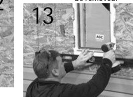
Place the Midframe in the opening. There is a tab on the backside of the flange that keeps the Window up and off the exterior sheathing. Center the Window left to right and install a 1 1/2" mounting screw in the bottom center of the flange closest to the tab. Level the window and install the rest of the mounting screws.
