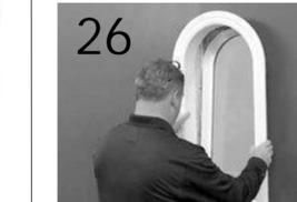
Place Interior Trim piece over Midframe jamb extension. The trim piece should fit flat against the wall.
