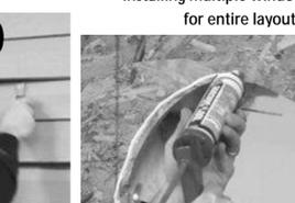
Apply a 1/4" bead of caulk around the entire edge of the window opening
