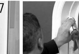
Using a caulking gun and the silicone supplied, fill the gap between the Mid-Frame and the Interior Trim at the midpoint of the jamb extension. Also fill any nail holes.
