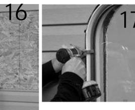
Replace any siding that was removed. There should be slight clearance between the siding and the protruding window. Use snips to trim siding if necessary.
