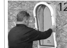
At the bottom of the window opening, draw a vertical line 3" long indicating the center point of the stud cavity. Place the Mid-Frame assembly into the opening. On the front of the flange at the bottom of the window is a vertical line. Align this molded reference line with the 3" line you just drew.
