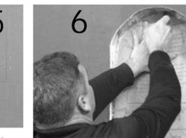
Cut away the insulation between the interior and exterior wallboard and remove. Use extreme caution and disconnect power if any wires are present.
