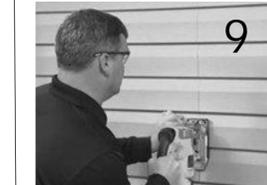
Using a reciprocating saw cut along the outline and remove the siding and exterior wall board. If installing multiple windows repeat as necessary.
