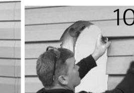
Remove all the siding around the window openings at least 6" from the opening. When installing multiple windows, the siding between the window openings must be removed.
