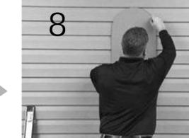
On the exterior side of the wall draw a level horizontal line at the bottom edge of the holes you drilled thru the exterior siding. Align your template to the lower horizontal line and drilled corner holes and transfer the template outline to the siding. Be sure template is level and plumb. If installing multiple windows repeat for entire layout.
