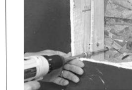
Using a 1/2" drill bit at least 7" long, drill a hole in each bottom corner through the outside wall board and through the exterior siding. These holes will be the bottom corners for the exterior cutting template. If installing multiple windows, repeat steps 1-6 for each window.
