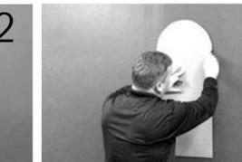
Using the template marked on the box, align the template between the stud lines and transfer the outline to the wall.
