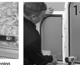
By aligning the saw tooth flanges of the Midframes, windows will align side to side within each stud cavity. Start installing windows from the center location and work your way out until all Midframes are installed.
