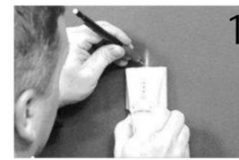
Using a stud sensor with an electrical wire sensor mark all stud positions. (You must have at least 14 between each stud.)
