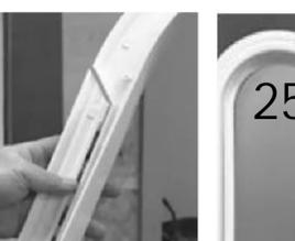
Interior Trim pieces also have guide ribs molded on backside. Use hand saw to cut Interior Trim to proper size. Sand edges if necessary to remove rough edges. If necessary refer to pictures at the end of instructions or website for detailed cutting information.
